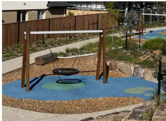
2a. EPDM Rubber- provides durable and colourful impact absorbing surface beneath play equipment
