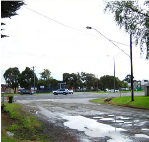
GLISMANN ROAD & PRINCES HIGHWAY EXISTING INTERSECTION
