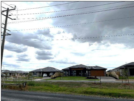
Plate 15 Residential development to the south of the land
